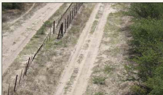
Damaged fencing southwest of the Onanke gate. It is believed that the majority of damage to this stretch of the veterinary cordon fence is caused by elephants.
